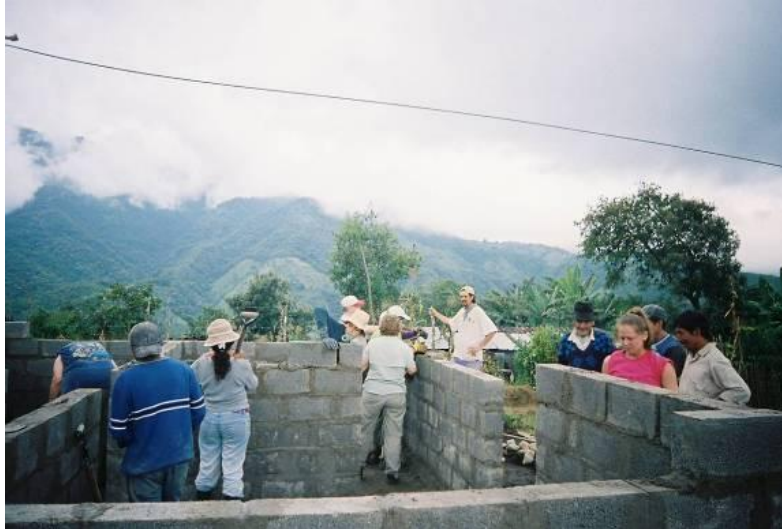
Work Project in Pucara
